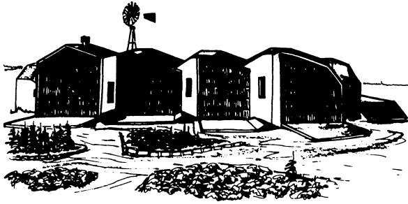
FIG. 17.2 The Baer house near Albuquerque, using water barrels mounted horizontally behind insulating panels which can be lowered during the day time to admit solar radiation, and raised again at night to conserve the collected solar radiation.
