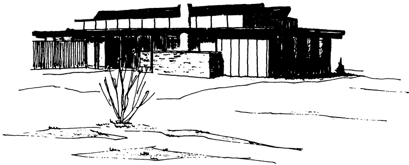
FIG. 17.7 The Löf house, erected in Denver in 1958. Two banks of overlapping glass collectors are used to warm air, which in turn heats gravel in two storage cylinders. Heating at night and during cloudy weather is accomplished by the stored sun-collected heat in the rock-filled cylinders.
