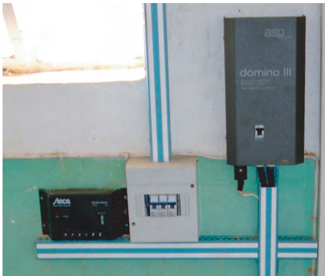
Figure 5.4 Charge controllers, MPPTs, main switches, inverters, fuse boards and other accessories on wall-mounted panels
