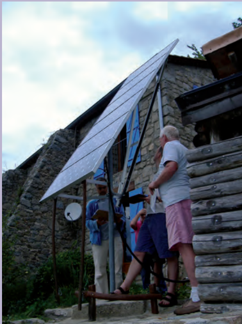
Figure 10.2 Seasonal angle adjustment of a fixed mount
