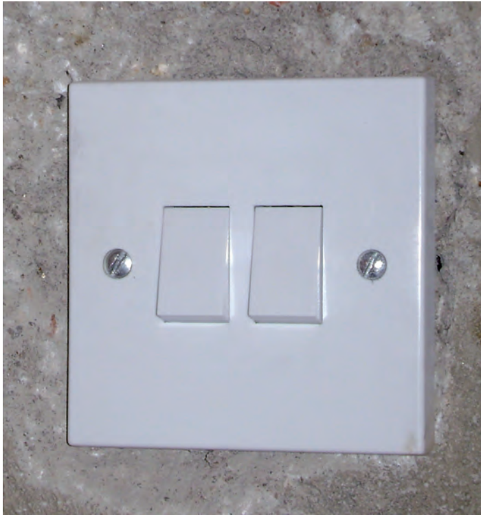
Figure 7.2 Common AC switches for lighting circuits
