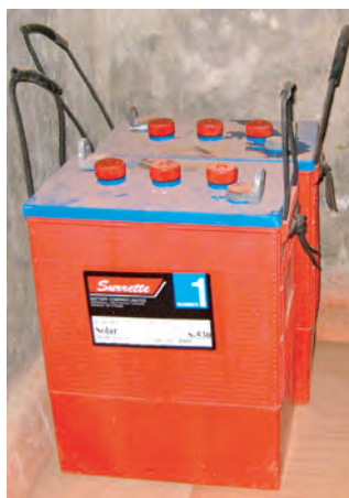
Figure 4.9 Types of battery: Sunset flat plate solar battery (top left); local Kenyan SLI batteries, not generally recommended but often the only option (top right); Hoppecke 2 volt cell, flooded, tubular plates, deep cycle, recommended for larger systems (bottom left); Surrette 6 volt batteries, deep cycle (bottom right)
