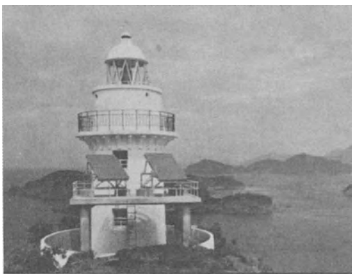
Fig. 1-3. Early Japanese installation. (Courtesy Sharp Corp.)
