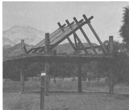
Fig. 7-12. Typical frame-mounted module installations. (Courtesy of Solarex Corp., JPL, and NASA Lewis Research Center.)
