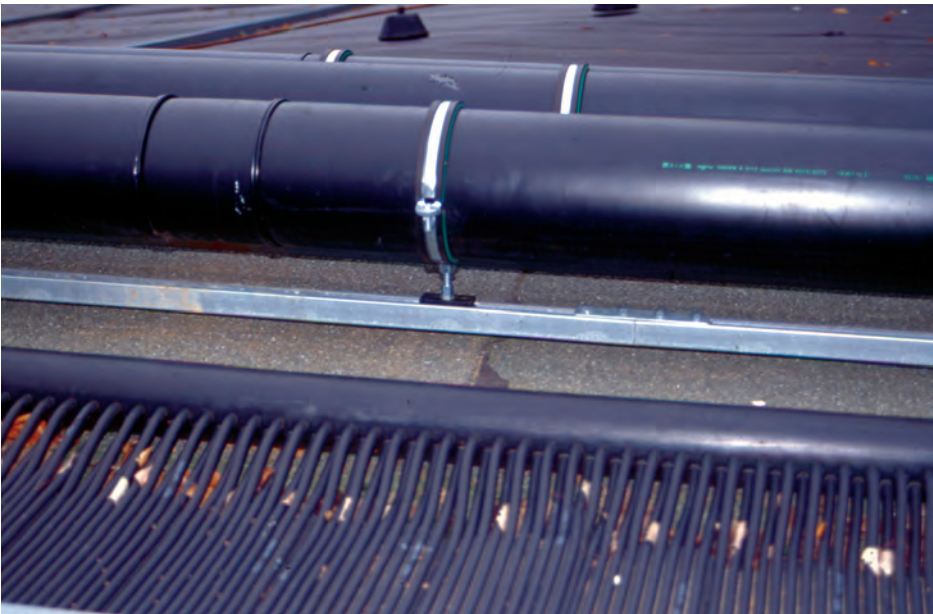
Figure 7.23. Example of sliding installation of pipe with anchor clamps
