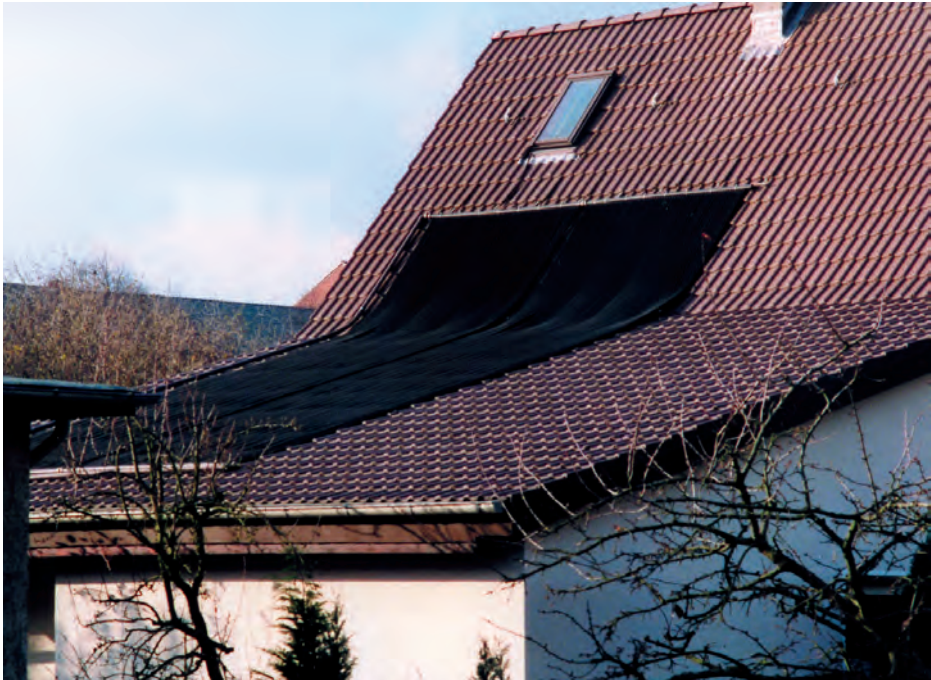
Figure 7.24. Private solar system for pool heating
