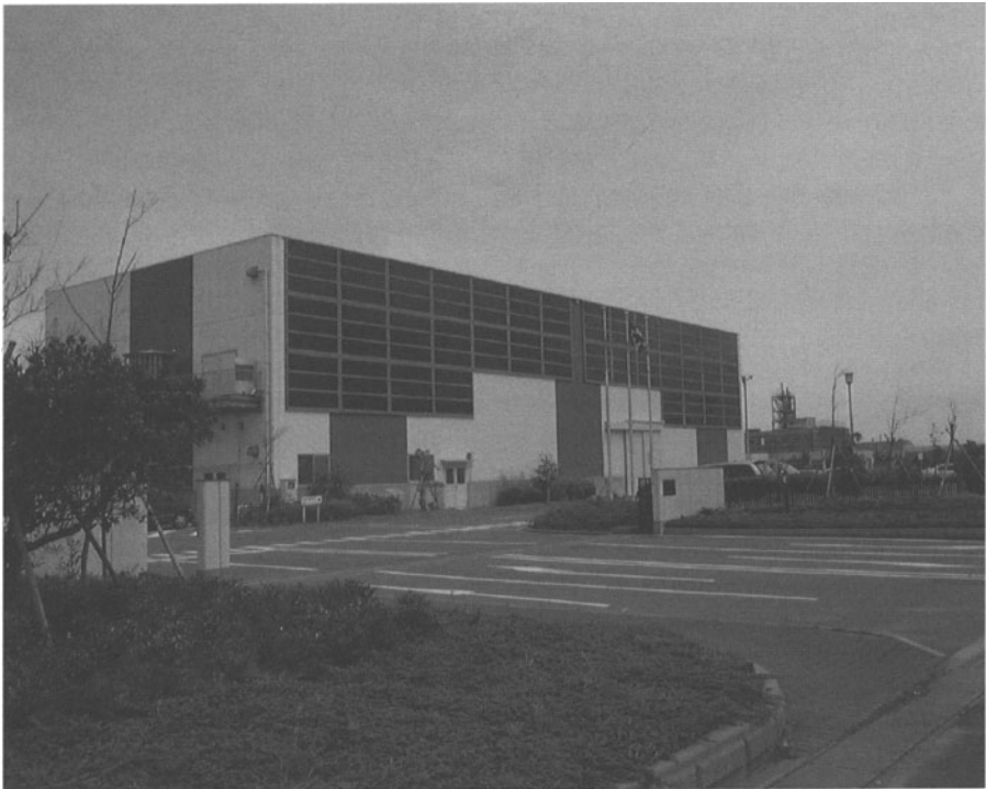
Fig. 6.15. Plant wall of Sumitomo Metal Mining Co. Ltd installing a-Si:H solar module integrated ACL panels with 10 kW capacity
