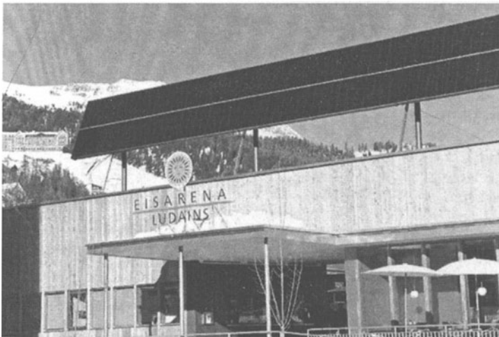
Fig. 12.22. Example of PV system (3) (CIS: Switzerland) (presented by FABRI SOLAR AG)
