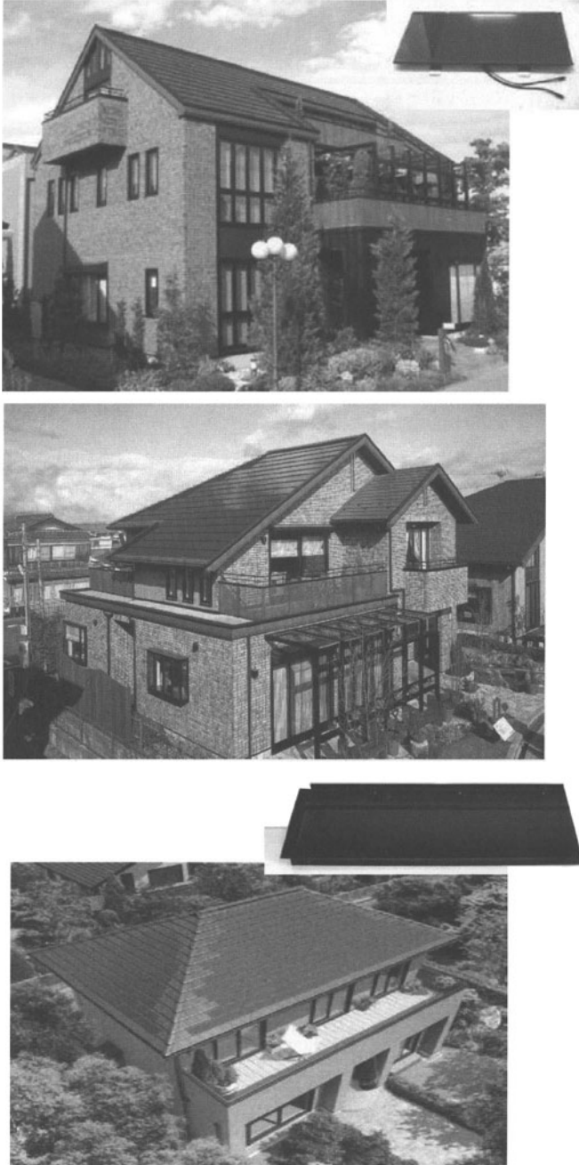
Fig. 9.13. Private houses with PV roofing tiles in Japan
