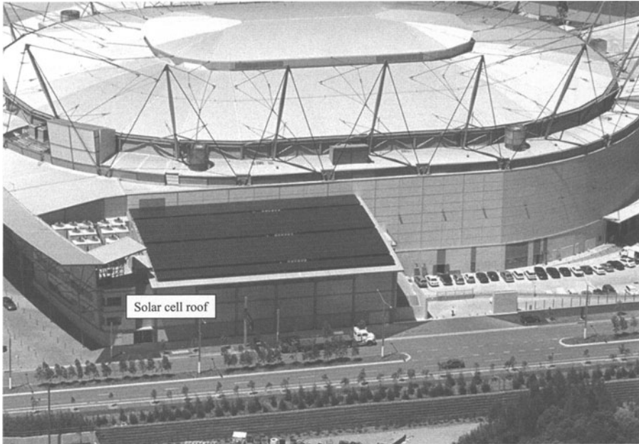
Fig. 7.9. Example of the installed roofing-material integrated PV modules
