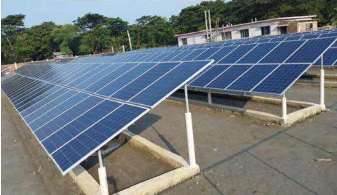
Example of beam type foundation
