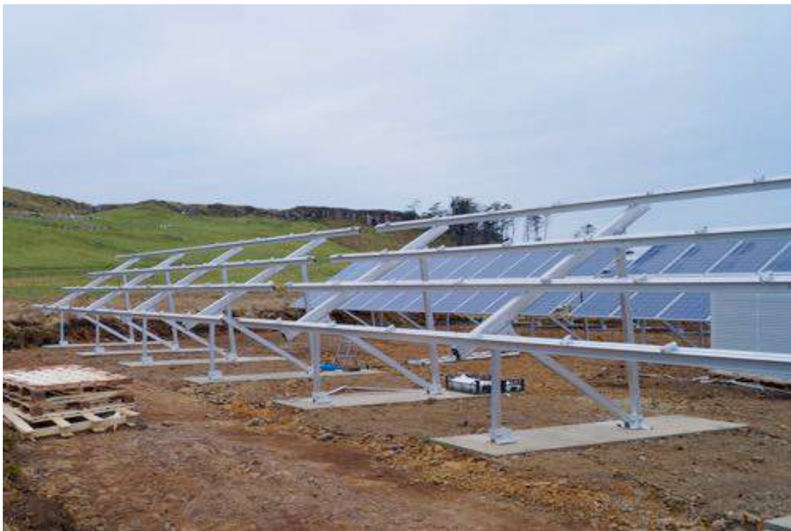
Example of slab foundation
