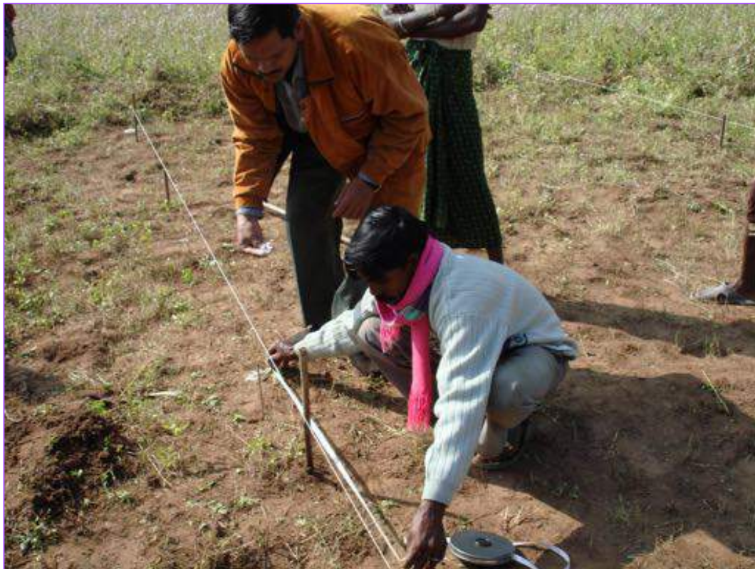
Aligning the locations for foundation for mounting structure
