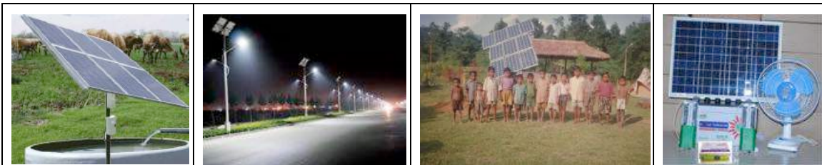
Examples of Standalone PV systems: solar water pumping system, street lighting, rural micro grid and solar home system
