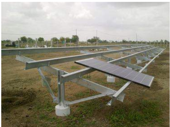
Example of block type foundation
