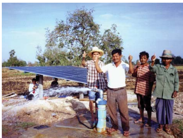
Fig. 7.14 “Historical” water pumping system in Thailand with ground-mounted framed a-Si modules. (courtesy of United Solar Ovonic)
