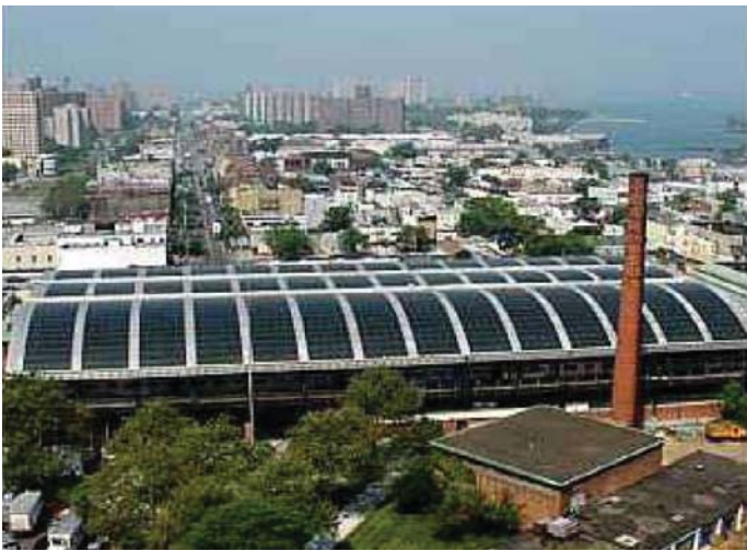
Fig. 7.12 Stillwell Avenue Train Station, Coney Island, New York City (credit SCHOTT Solar AG).
