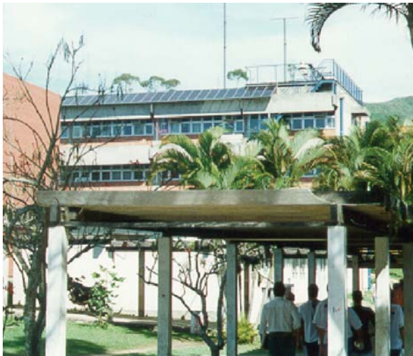
Fig. 7.8 Front view of the 2-kWp a-Si thin-film PV installation in Florianópolis, Brazil. (with permission [Rüther-1998])
