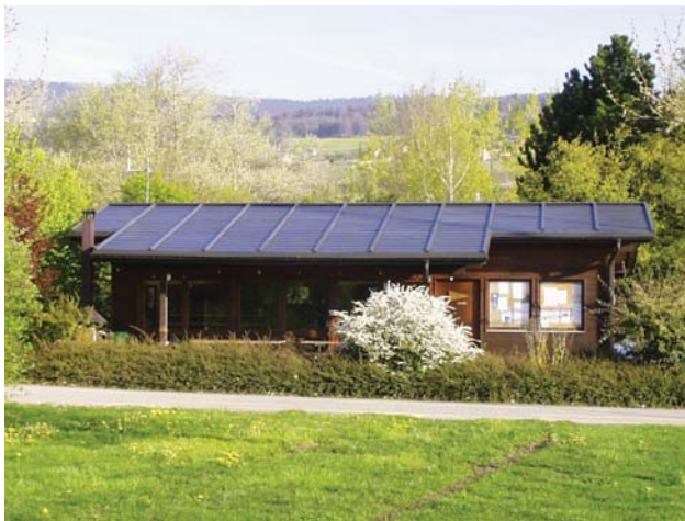
Fig. 7.6 Front view of PV roof “La Galère”, Auvernier, Switzerland (with permission [Shah-2004]).
