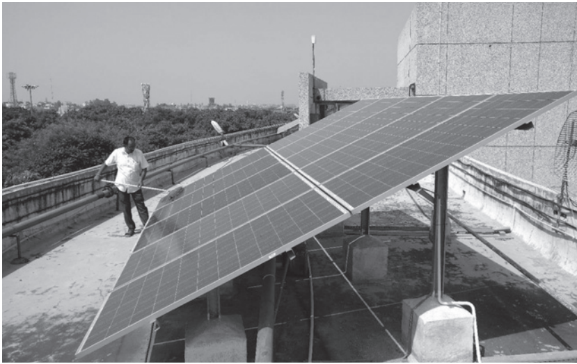
FIGURE 13.2 Maintenance of PV arrays.
