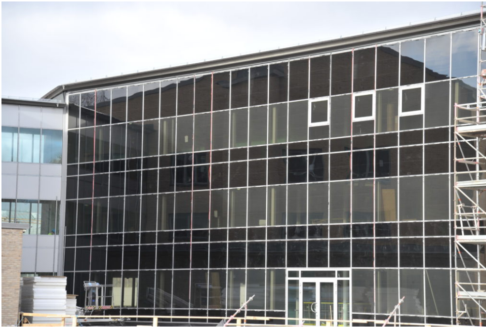
Figure 1: SolTech windows built into the facade of Vallaskolan by Skanska
