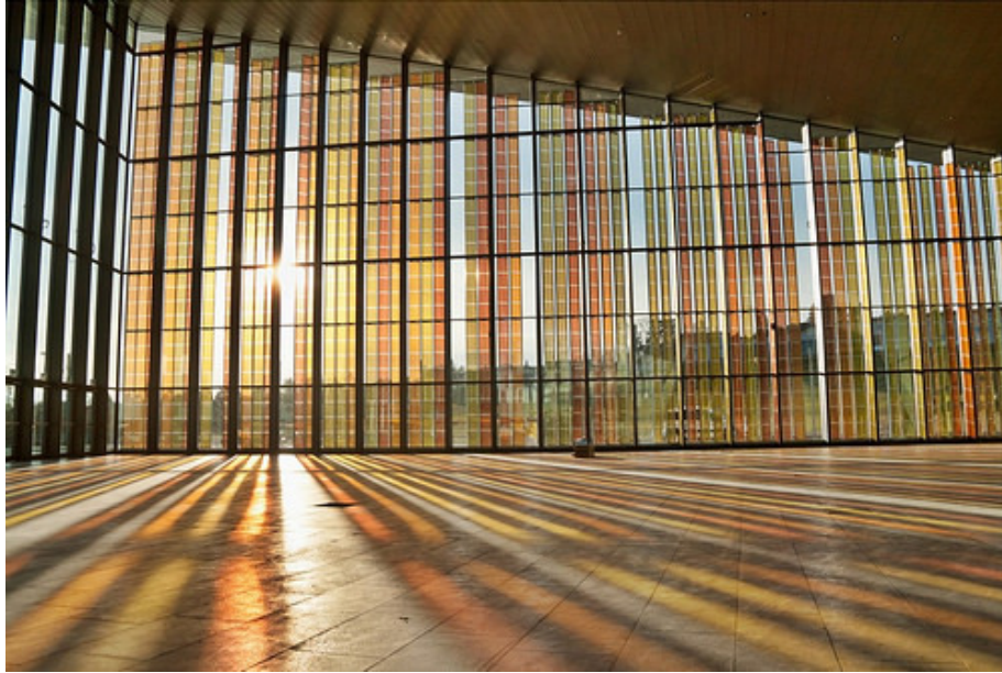
Figure 2: School of technology in Lausanne with dye-sensitized solar cells as semi-transparent windows
