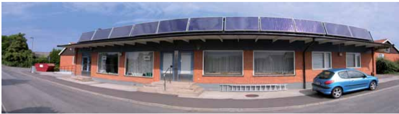
Figure 2.19 Building integrated photovoltaics in Bunkeflostrand in Malmö, Sweden. (Photo: Schüco Internation KG).
