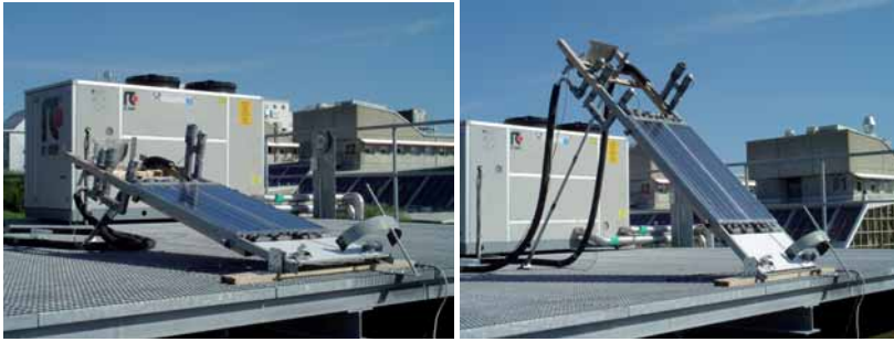
Figure 3.4 A solar collector mounted on the roof of the EBD Laboratory and adjusted to different tilt angles.
