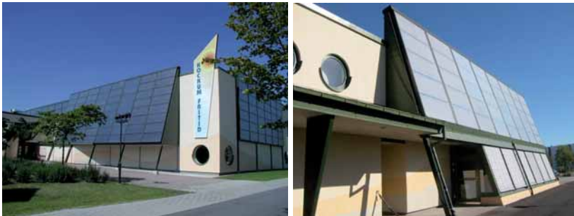
Figure 7.1 The large façade-integrated collectors at Kockum Fritid in Malmö. (Photo: Martin Råberg, Grontmij).
