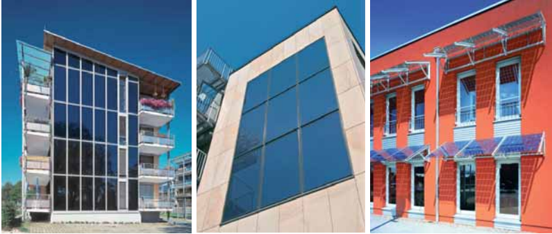
Figure 2.18 Building integration of solar thermal collectors in façades (to the left and in the middle) and of photovoltaics in solar screens (to the right). (Photo: Schüco Internation KG).
