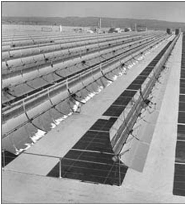
FIGURE 5.2 Concentrating Solar Power System: Trough Style, Mojave Desert, California
