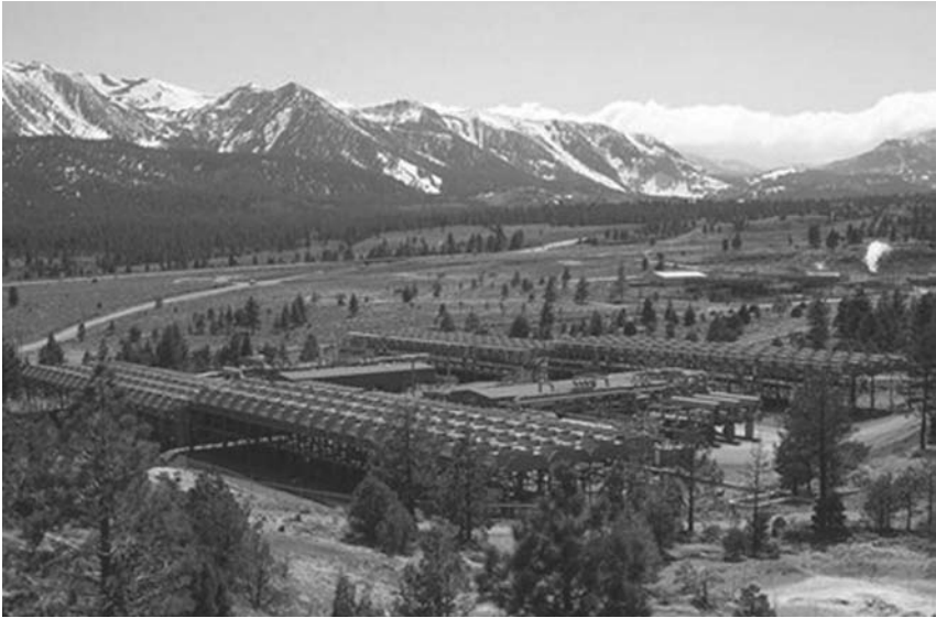
FIGURE 3.1 Mammoth Pacific Geothermal Power Plant located in the Sierra Nevada Mountains, California, 28 megawatts Source: Geothermal Resources Council and National Renewable Energy Laboratory, Pix Number 10991, http://www.nrel.gov/ .
