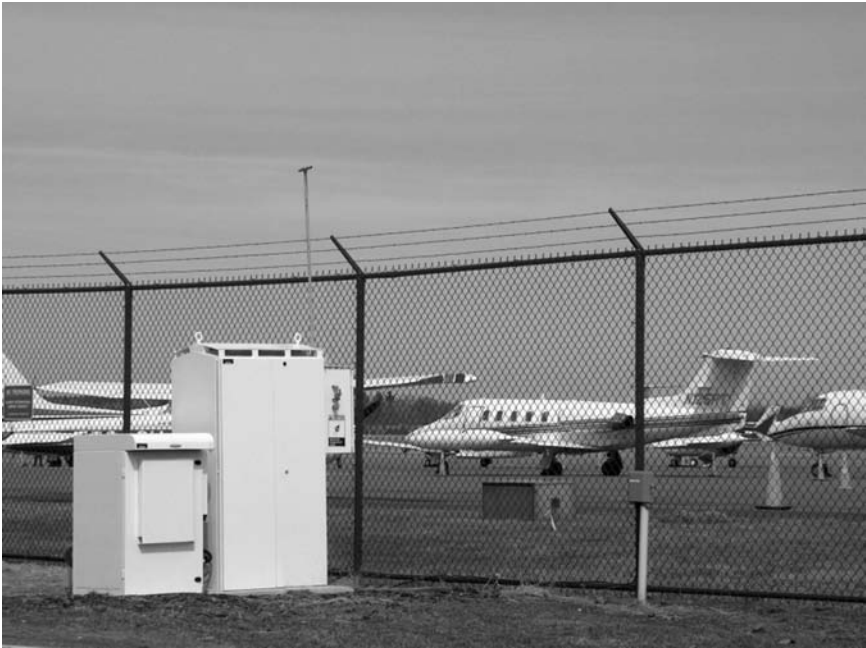
FIGURE 7.2 PEM Fuel Cell: Remote Application
