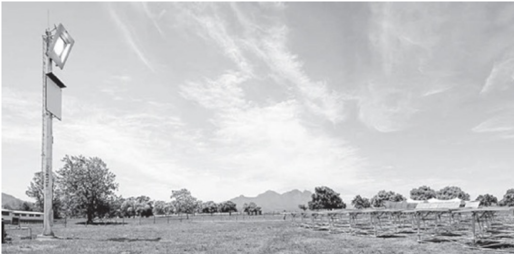
The Helio100 trial installation in South Africa.
