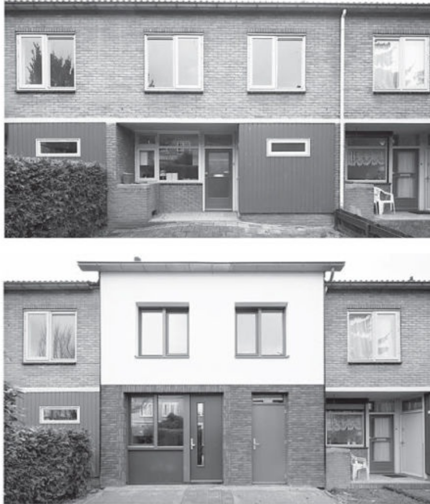
A Dutch Energiesprong house, before and after refurbishment.
