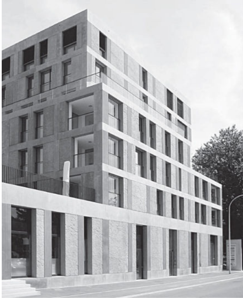
Heliatek film installed on a concrete building. The ultra-thin films can be mounted on glass or concrete to generate power.
