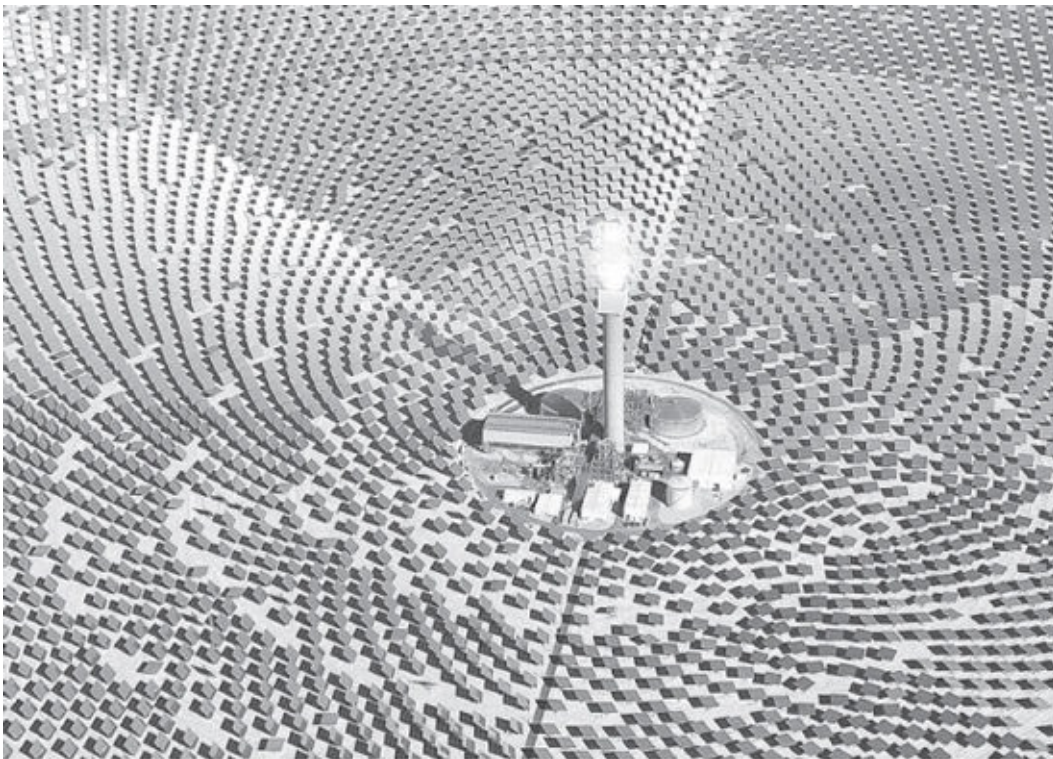
The innovative Crescent Dunes CSP plant in Nevada.
