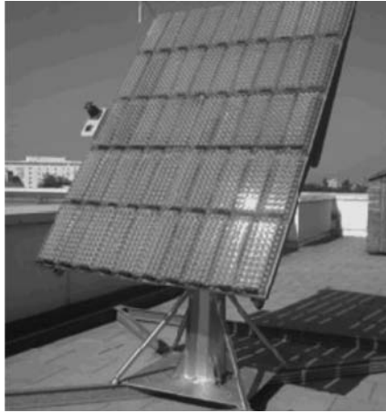
Figure 5.13 Photograph of the grid-connected CPV system using FLATCON®-type modules on top of the roof of Fraunhofer ISE. In Europe, this is the first CPV demonstration system using III-V cells (Source: Bett et al. 2003, reproduced with the permission of Dr. Andreas Bett)
