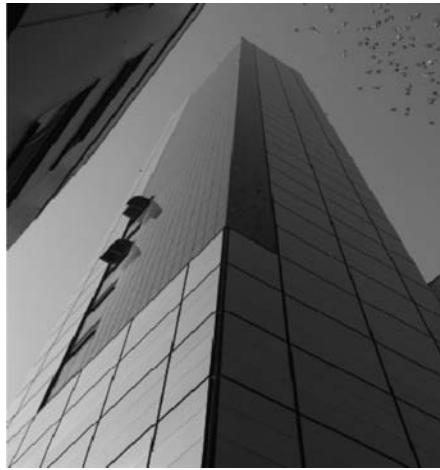
Figure 3.9 Grain silo 'Schapfenmühle' on the outskirts of Ulm, Germany. 1306 CIS modules from the Würth Solar pilot plant with a nominal installed power of 98 kWp are integrated into the façade (Source: Powalla & Bennet 2007, Hindawi Publishing Corp., Copyright © 2007 M. Powalla & D. Bonnet)
