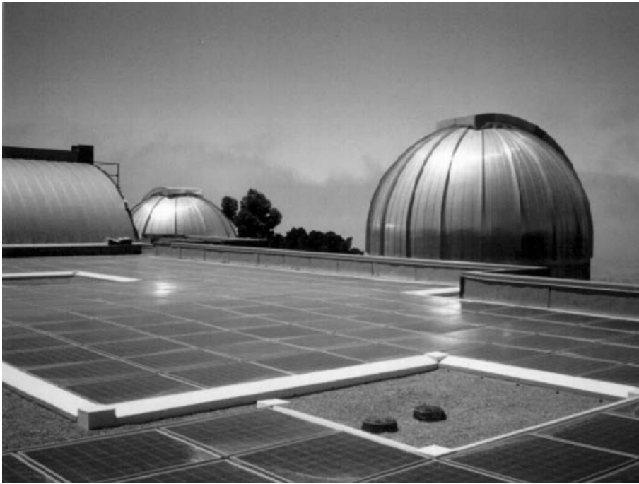
Figure 14.1 Powerlight foam solar PV collector roof tiles.
