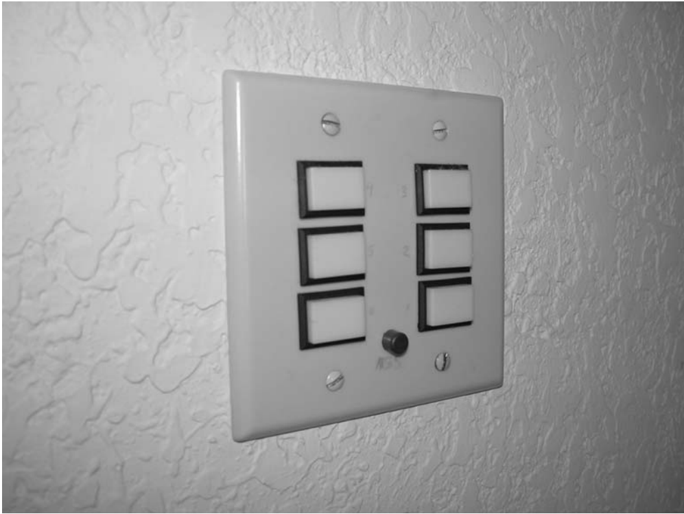
Figure 13.7 Localized special function toggle switches.
