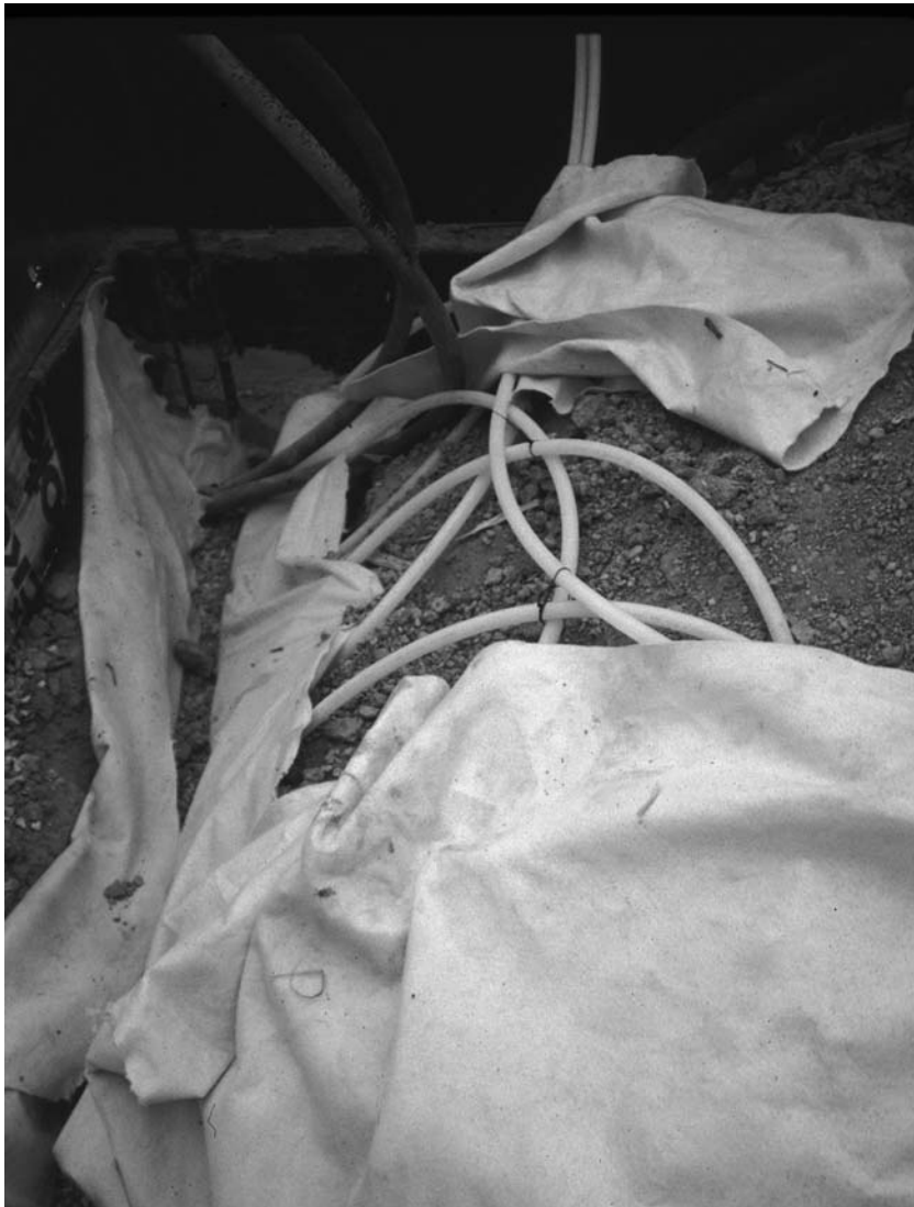
Figure 7.7 Photograph showing installation of ground coils.
