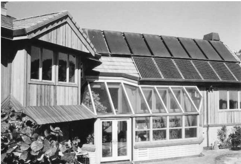
Figure 1.5 Completed Berkeley Solar house configuration.
