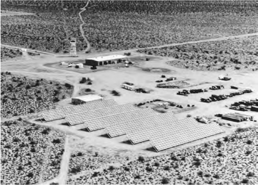
FIGURE 12-6 A 300 kW photovoltaic-diesel hybrid system in Superior Valley, California. (Source: ASE Americas Inc., Billerica, MA. With permission.)
