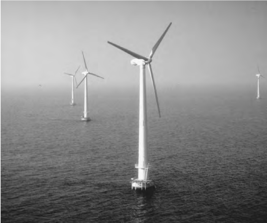
FIGURE 16-6 Vindeby offshore wind farm in Denmark. (Source: Vestas Wind Systems, Denmark. With permission.)
