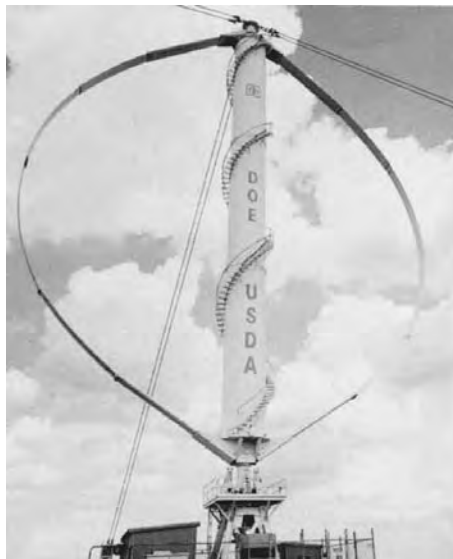
FIGURE 4-2 Vertical axis 34-meter diameter wind turbine built and tested by DOE/Sandia National Laboratory during 1994 in Bushland, Texas.
