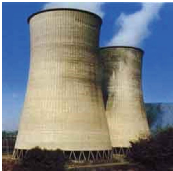
Fig. 2.17 Cooling towers in a CSP plant
