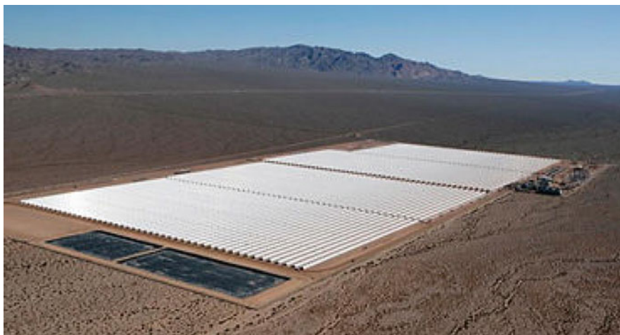
Fig. 2.16 Nevada Solar One CSP plant
