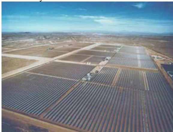
Figure 3: Picture showing five 30 MW e units of the solar parabolic trough plants at Kramer Junction, California (source Quaschnig and Trieb 2001)
